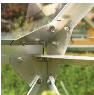
Roof braces, corner plates and side braces for additional strength
